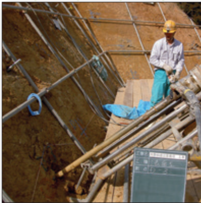
切土補強土工
