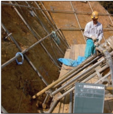
切土補強土工
